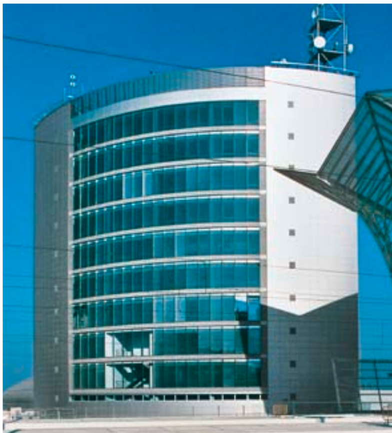
Portugal Telekom, Lisbon, Portugal
