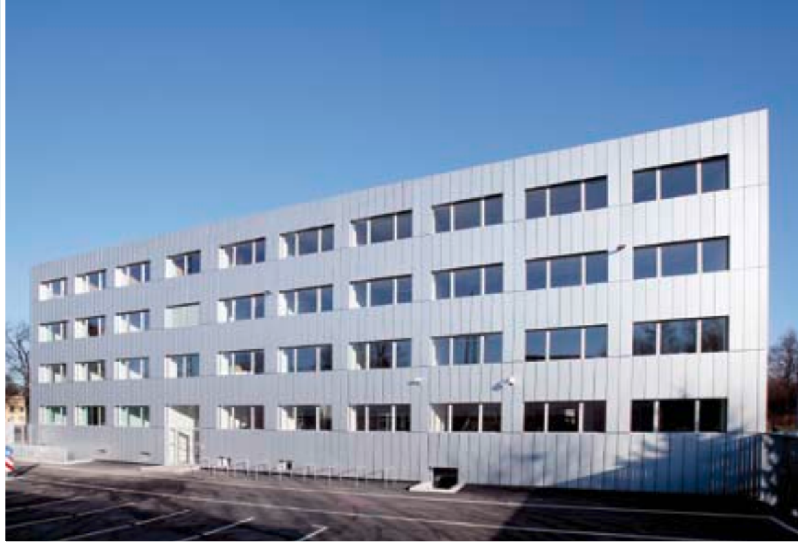
Police Station, Chemnitz, Germany
