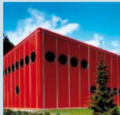
Factory building Dial-Norm, Kirchberg, Switzerland
