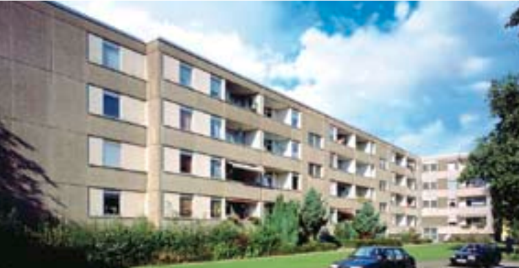
Residential buildings, Dortmund, Germany, before
